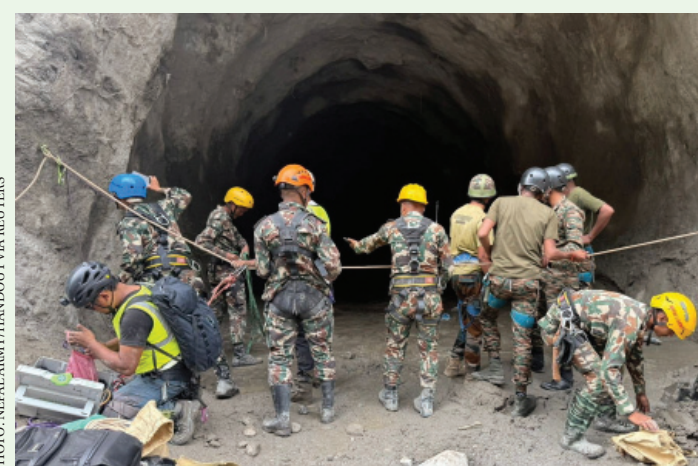
Nepal army soldiers work during a search and rescue operation outside a tunnel near the Hydropower Project sites, following deadly flash floods and mudslides, in Rasuwa district, Nepal, in this handout obtained by Reuters on September 1, 2026.
